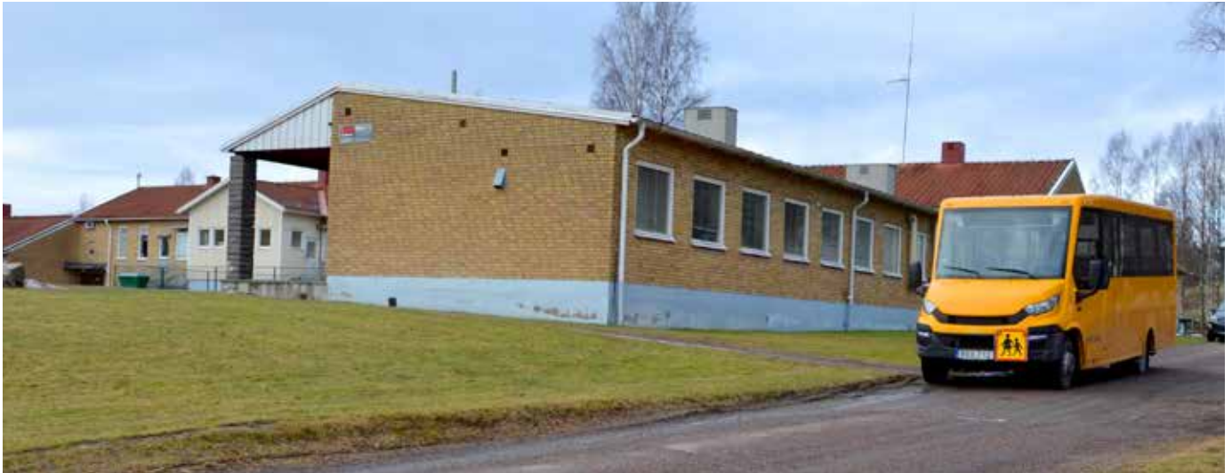
Edane Elementary school
