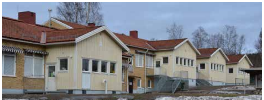
Edane Elementary school
