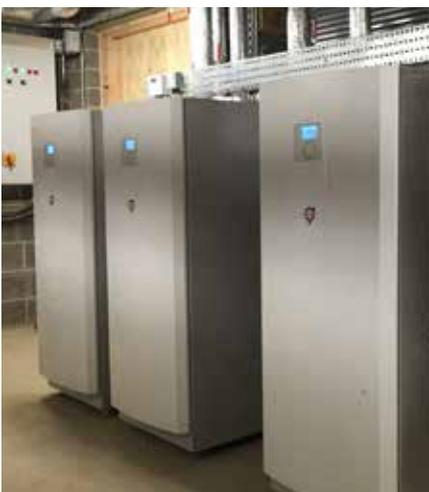
Thermia Robust ground source heat pumps
