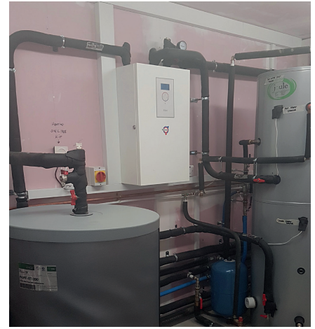
Thermia Atec Plus unit and a 180 litre domestic hot water cylinder
